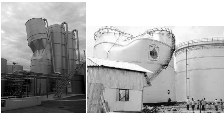
Figure 1: Examples of tank collapse
